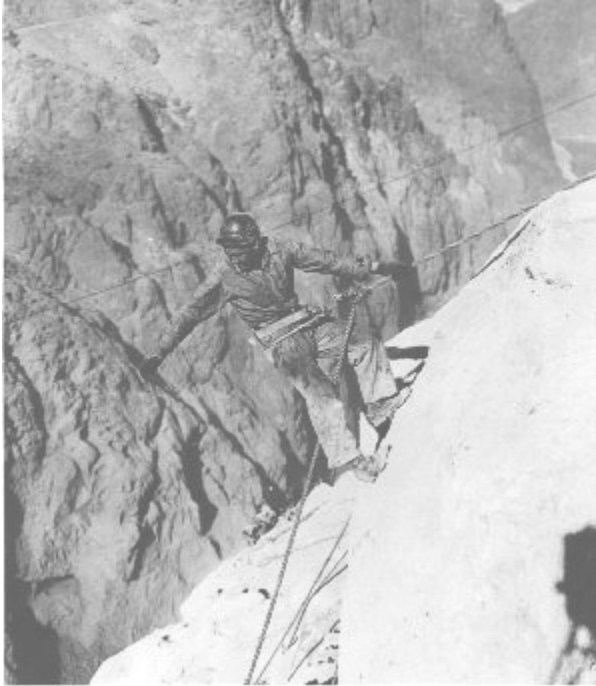
Figure 1-5. High scaler on Hoover Dam
